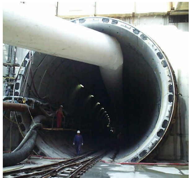
Application in tunneling
